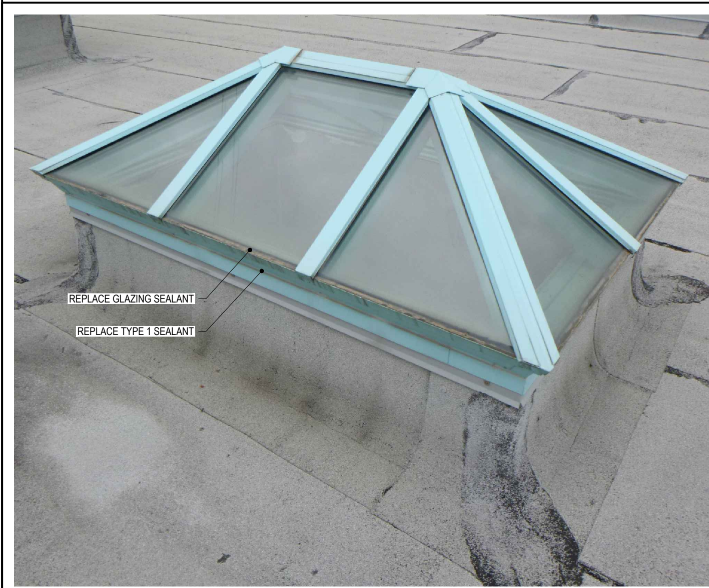
5 TYPICAL SKYLIGHT REF: SCALE: NTS
