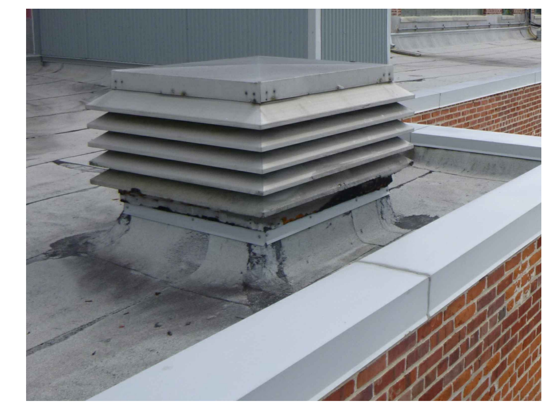
5 LOUVERED PENTHOUSE REF: 1/A-010 SCALE: NTS
